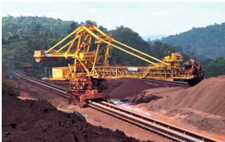
Iron ore storage area at Carajás
