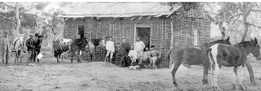
Chagas, Penna and Motta (seated, from right to left): this is the house where the doctor first became acquainted with the “barbeiro,” in 1908
