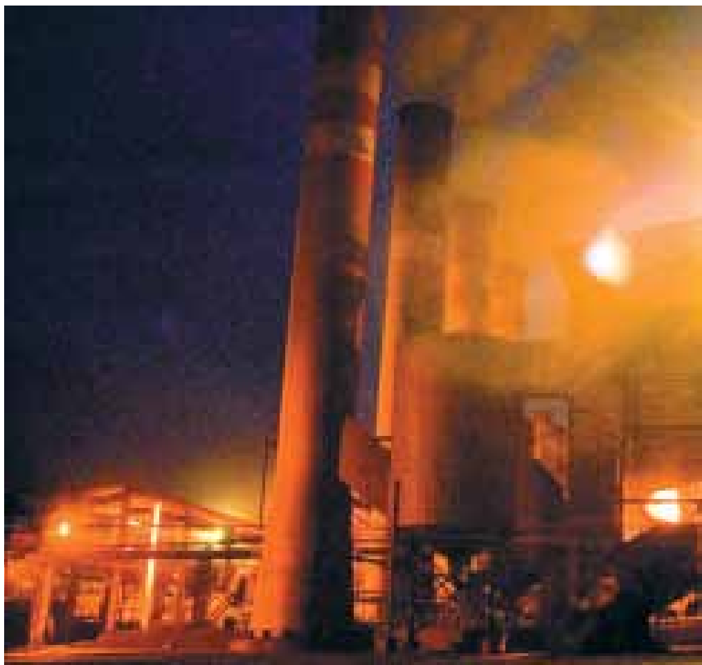
Boilers at the Santa Elisa Plant in Sertãozinho (SP): electricity production from sugarcane bagasse
