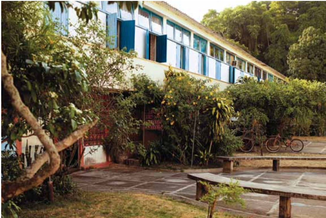
Paquetá housing project in Rio (left), built in 1952, and a building from the early years of Brasília: past attempts to harmonize housing projects and their environments
