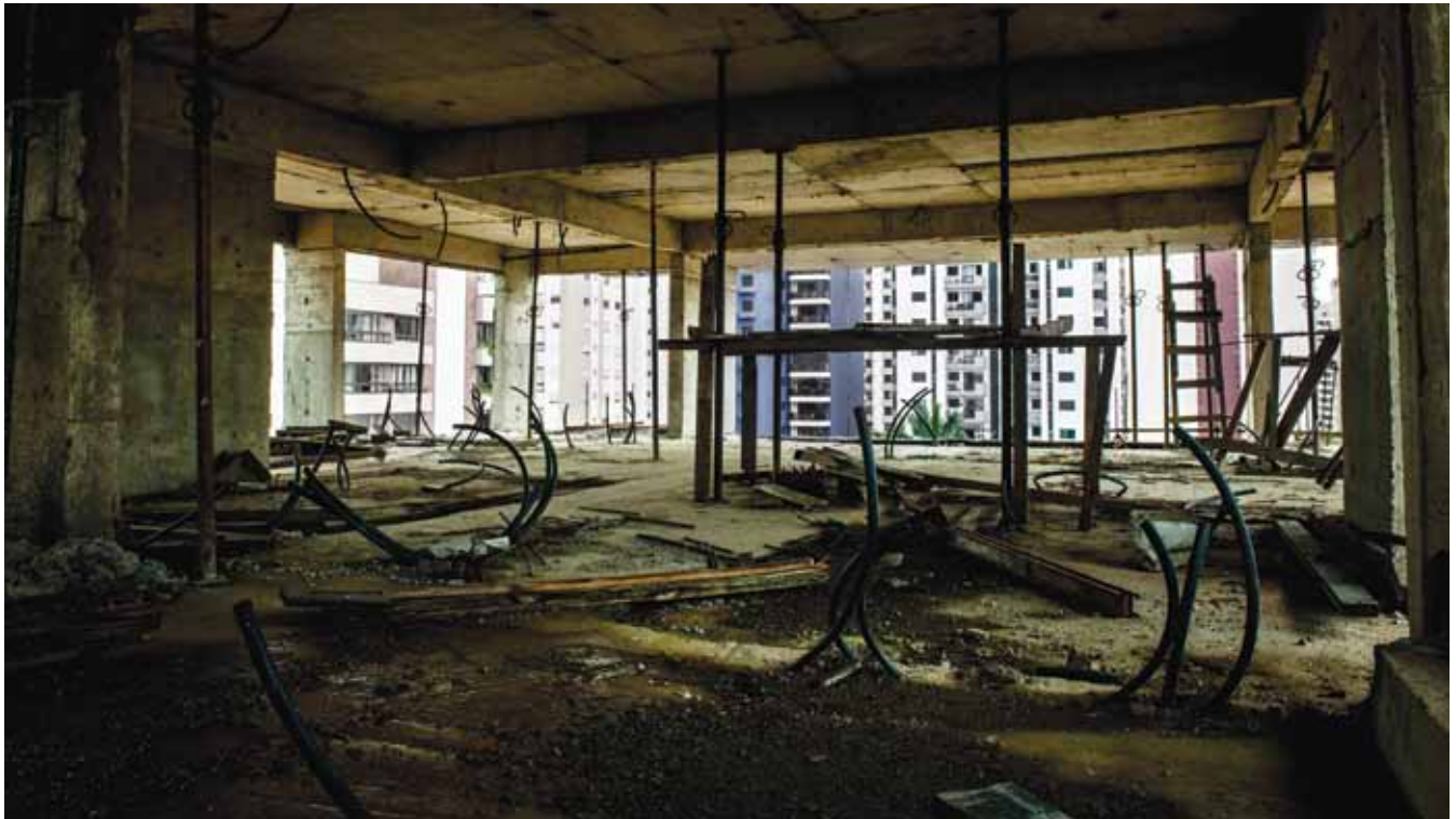
In the foreground, the skeleton of a building in Vila Leopoldina in the western zone of São Paulo. In the background, new buildings that rose during the real estate boom of the early years of this century
