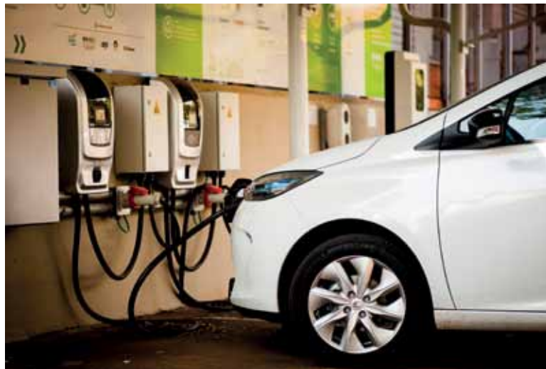
Electric Vehicle Laboratory in Campinas run by the CPQD and CPFL Energia: evaluating recharging outlets
